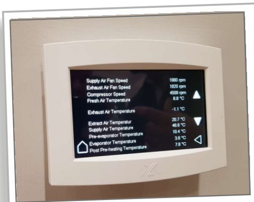
HPV Series main controller showing fan speeds, fresh air, exhaust, extract and supply temperatures.
