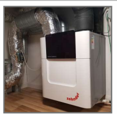
Zehnder Q350 providing some heat recovery ventilation along with some space heating from an inline duct heater
